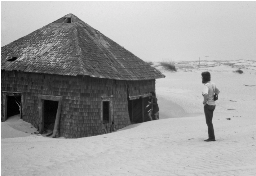
Exploring one of the early beach structures at False Cape.
