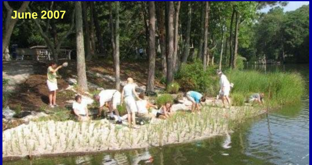
After - fiber logs + sand fill + plants
