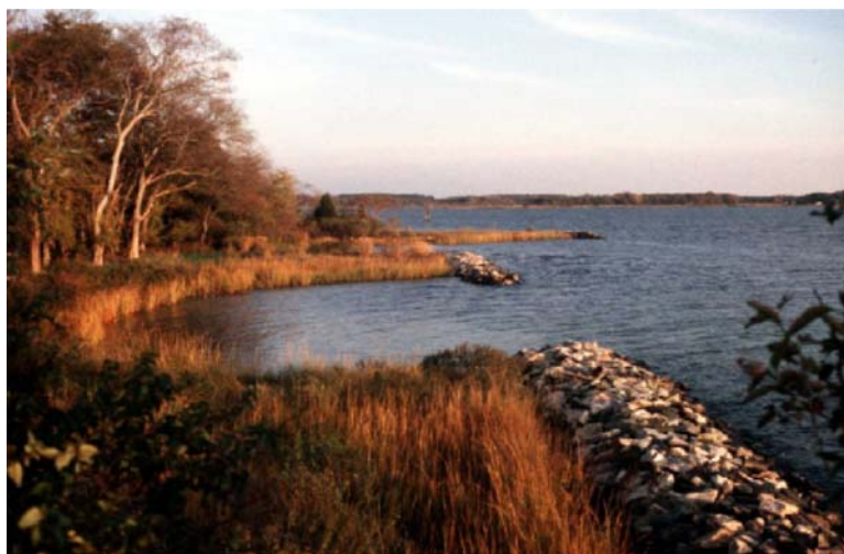
c. Breakwater and sill project after 5 years
