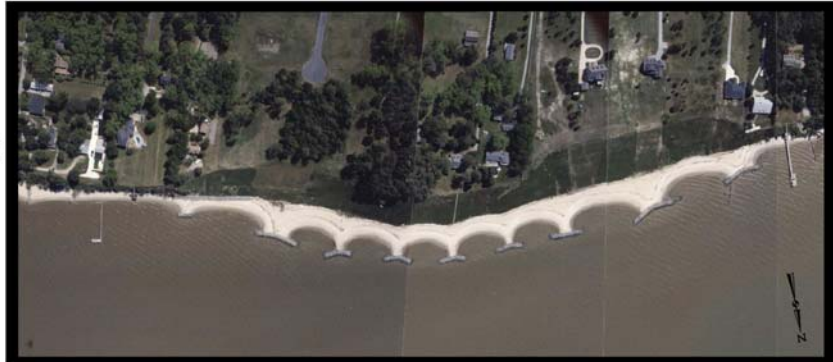
VanDyke Project Two Years After Construction 1999
