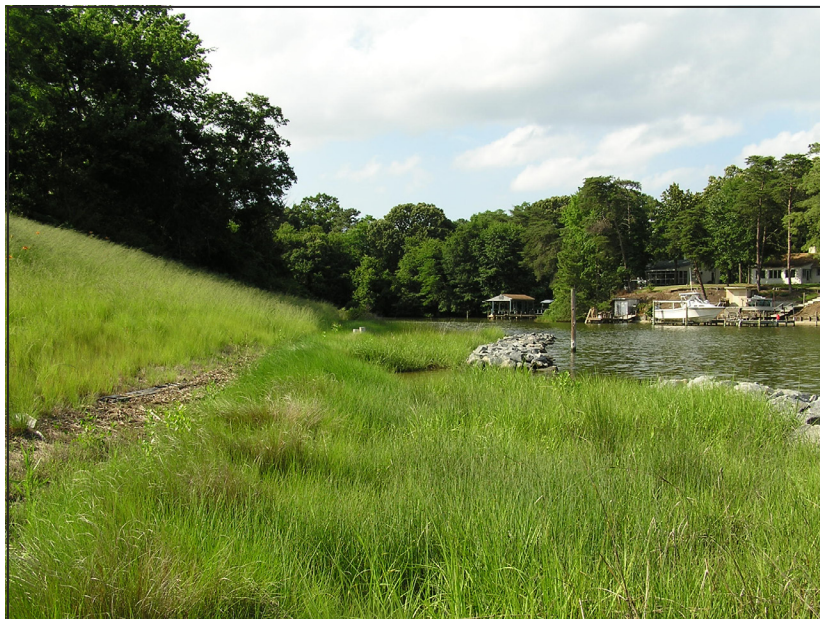
Shoreline best management practices protect the bank and create habitat.
