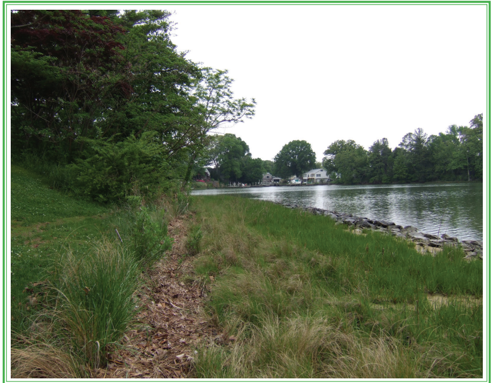
A marsh sill and planted marsh at Hull Springs Farm in Westmoreland County after three growing seasons and two major storms.
