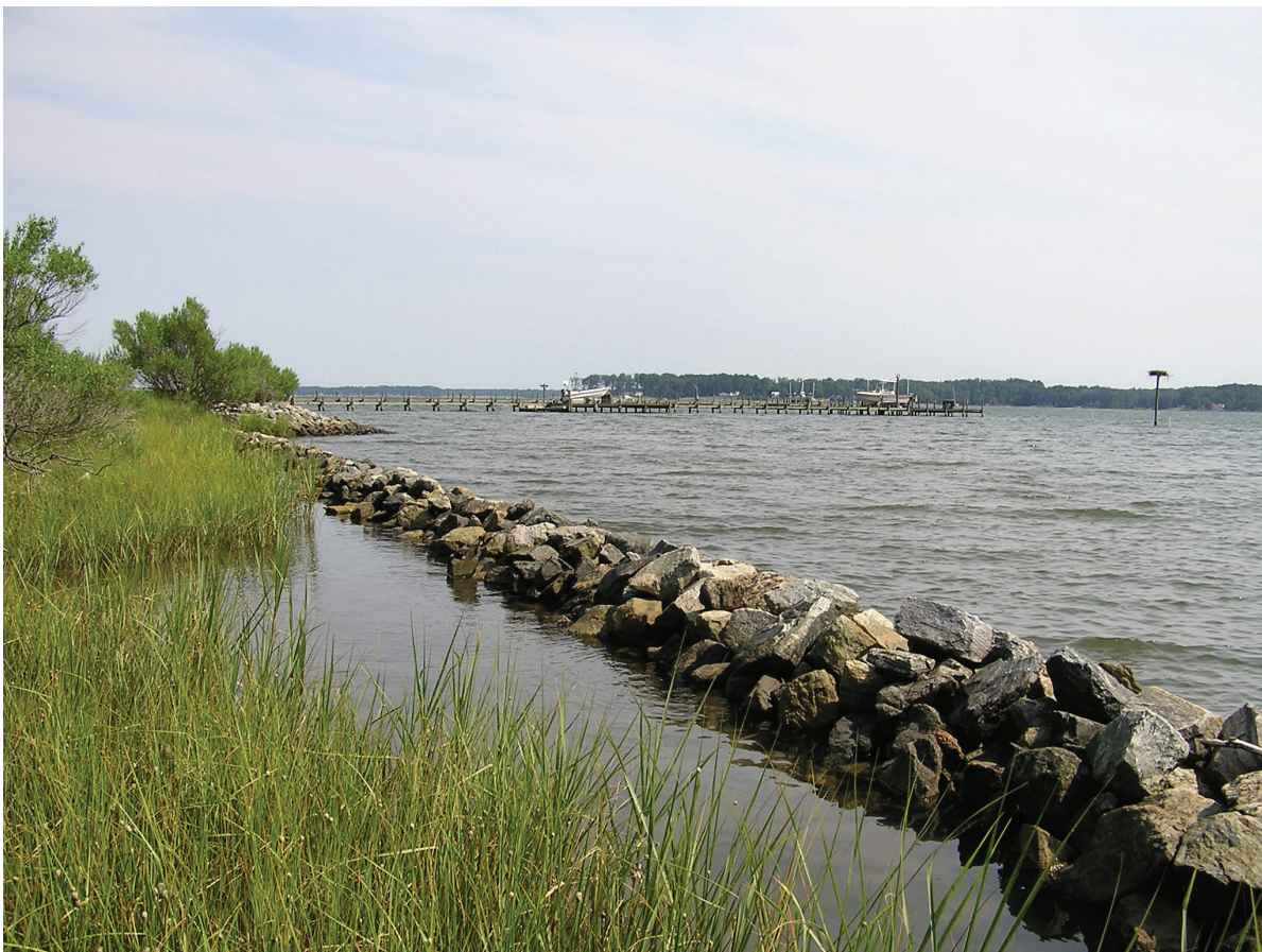
Calm water in the lee of a marsh sill on the Rappahannock River in Middlesex County.
