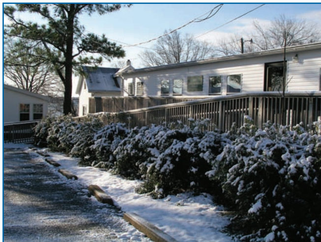
A portion of the CCRM complex
