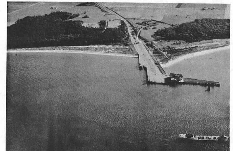
Plate 1 Kiptopeke Ferry Pier
