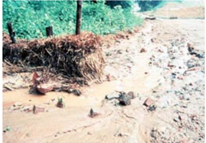
Figure 12. Sediment-laden run off.
