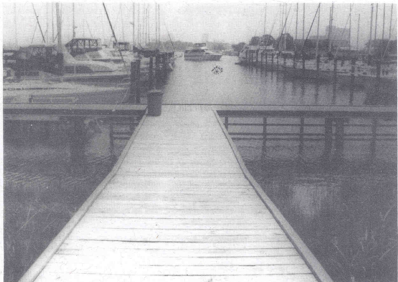
Access to navigable water should be achieved by piercing across wetlands rather than dredging and filling.
